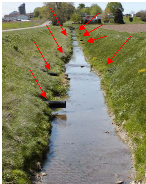
Field tiling along newly constructed ditch
