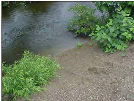
Figure L-13: Gravel Sloughing off into Stream
