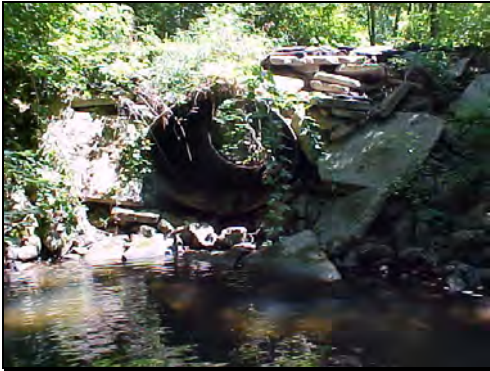
Figure L-3: Culvert Directly Upstream of CC3
