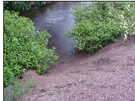
Figure L-14: Gravel Pile Along Streambank
