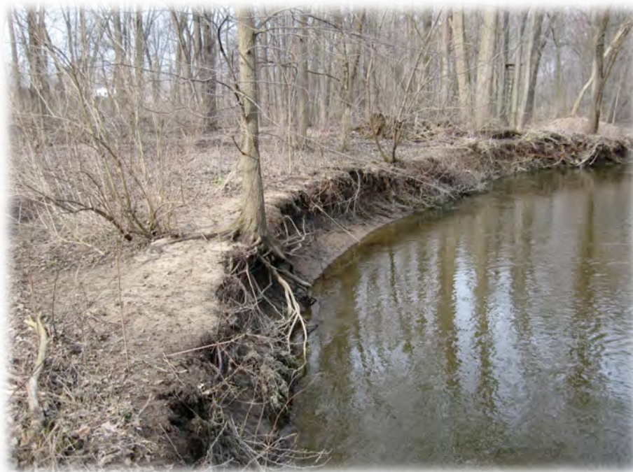
Pigeon Creek; Streambank Erosion
