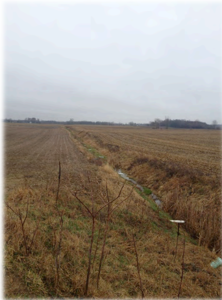
Drainage Ditch; Upper Pigeon Creek Watershed
