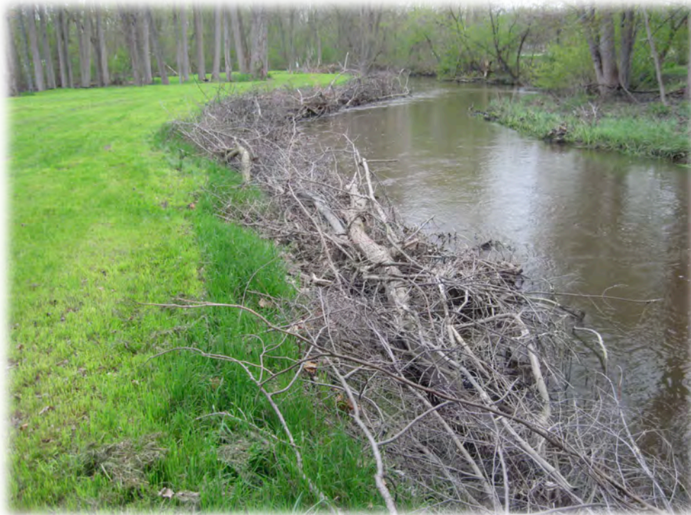
Pigeon Creek; Streambank Stabilization
