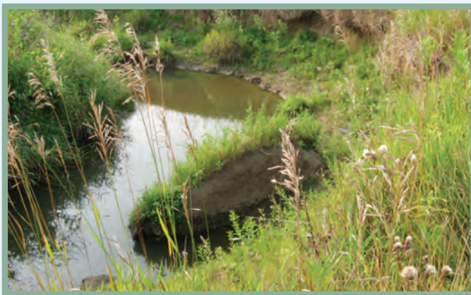
Figure 1. A: A trapezoidal ditch in Indiana with bank erosion and mass bank failures.
