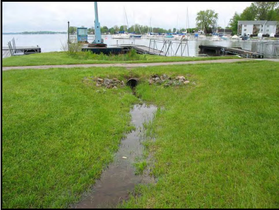
Figure 8. Ditch at public access site
