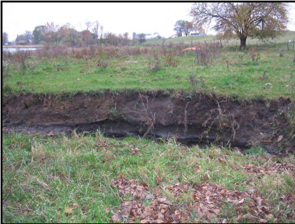
Figure 34. Streambank erosion occurring within a Wawasee Area Watershed stream.
