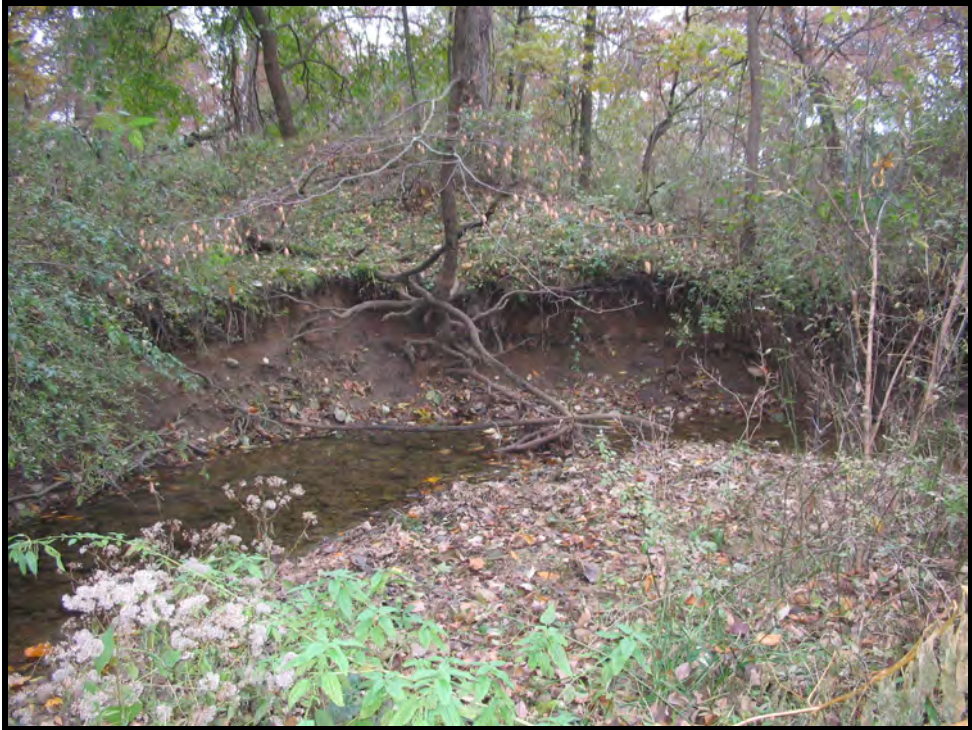
Erosion along tributary to Village Lake.
