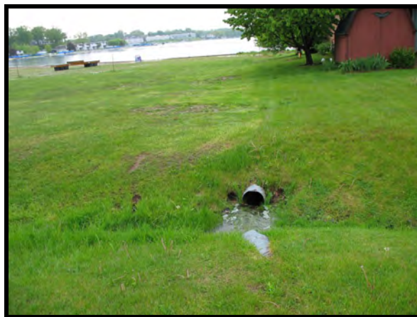
Figure 9.4b. Downstream of road.
