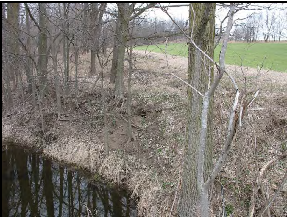
Minor erosion along the Ritter Branch (tributary to Harper Lake).
