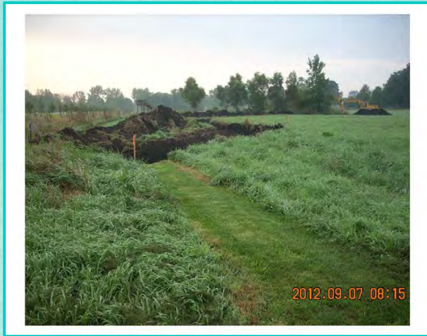
Diversion Channel Construction
