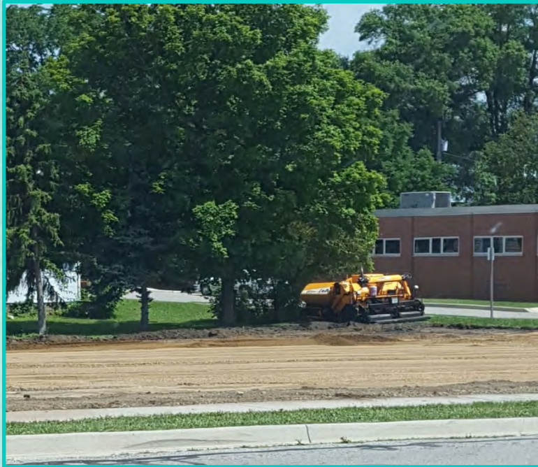
Parking Lot Construction
