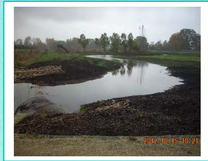
Diversion Channel Completion
