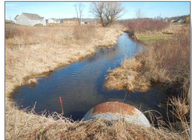
Perched culvert on Cobus @ CR 2
