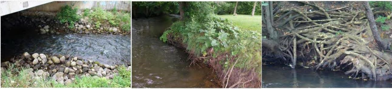
**Figure 17: Burr Oak Road Bridge, erosion and scour pools created from increased water flow**
