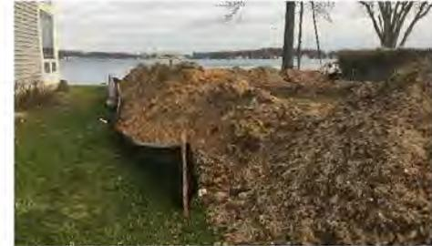
**Don't use silt fence as a retaining wall for stockpiles of soil!**
